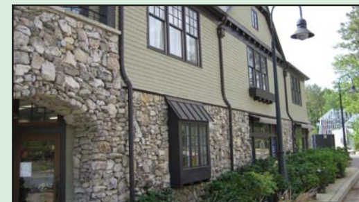
Exterior building materials should convey a natural and somewhat rustic feel with the use of stone, wood shingles, and similar materials. Lighter materials should always be located above heavier materials.
