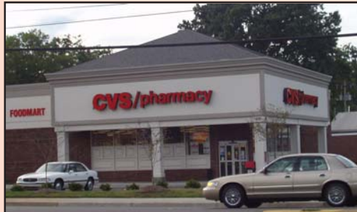
The Town Center may have pitched roofs, but they should feature overhangs rather than the roof edge being encased in a large cornice, as occurs above.
