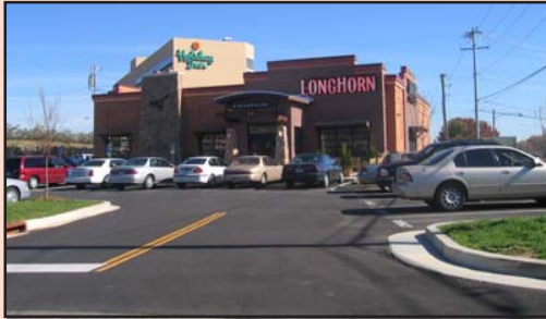
Building heights in the Town Center should not exceed two-and-a-half stories. The front setback above is too deep, and parking should not be in the front.
