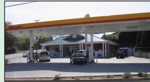
Existing Gas Station
