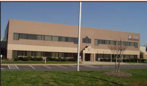
This building facade's uninterrupted plane fails to achieve the massing that is appropriate for a human-scaled and pedestrian-friendly environment. It also has a horizontal orientation rather than vertical bays.
