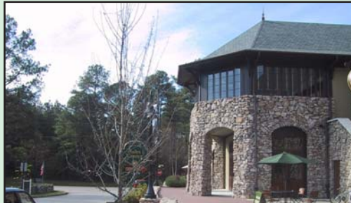
Buildings in Lookout Mountain's new Town Center should have either pitched or flat roofs. Pitched roofs should have a moderate to steep slope.
