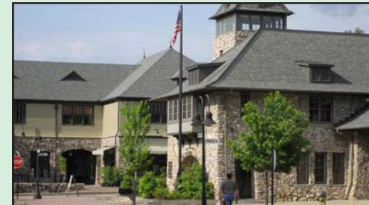
Flat roofs should be screened with a parapet facade along their street frontage. Dormer windows are also encouraged if appropriately proportioned.
